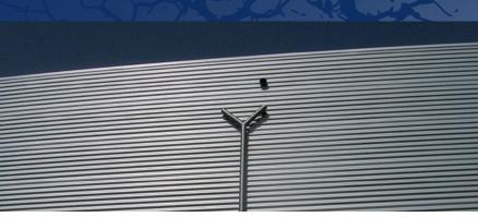
This sandwich panel with sinus corrugated external sheet and hidden fixing is a great esthetical option for modern facades by giving them a lively touch with its original wave design. The highly heat insulating CFC and HCFC free polyurethane rigid foam core suits best for today's requirements for thermal insulation and moisture protection. A non-displaceable sealing strip foamed into the longitudinal joint procures resistance to driving rain
