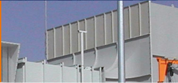
With its perforated internal sheet the Hipertec® Roof Sound panel contributes drastically to the improvement of sound insulation and sound absorption where applied. Designed particularly for ceiling application it may also be used as external roof in specific cases, including unheated premises. However for heated or moist areas the use of Hipertec® Roof Sound panels is not recommended since the internal sheet has no vapour barrier.
