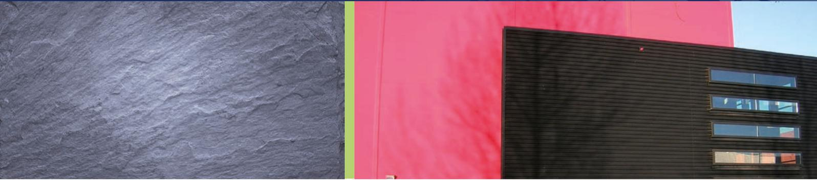
The Superwall® HF sandwich panel with microprofiled external steel sheet, non-combustible rock wool core and joint geometry for hidden fixing is suited best to meet today's sophisticated requirements for high-quality facades. The panels can be placed vertically or horizontally and, depending on the insulation thickness, may reach a fire resistance up to 90 minutes. Additionally Superwall® HF panels show excellent acoustic insulation behaviour as well. For building exposed
